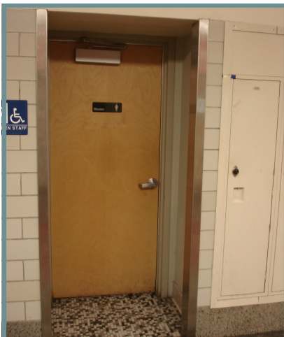
Door requiring power assistance
